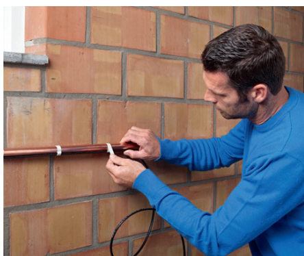
Attach the heating cable to the pipework.
