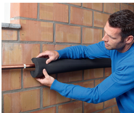
Cover the pipe and the heating cable with insulation.
