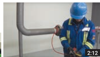
nVent RAYCHEM E-100 End Seal Kit Installation
