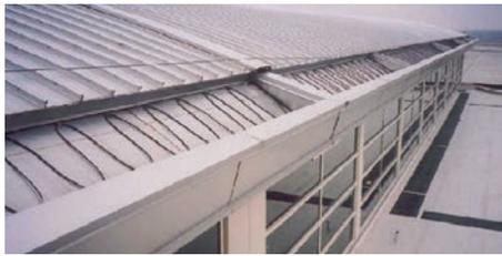
nVent RAYCHEM **roof & gutter de-icing systems** are advanced, high performing and often specified for buildings and offer reliable state-of-the-art connection kits and control systems. These systems are ideal for commercial buildings in light to heavy snow load areas.
