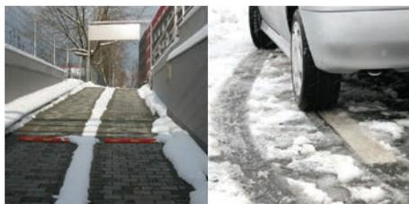
nVent RAYCHEM **surface snow melting systems** keep ramps, access ways and footpaths free of snow and ice.
