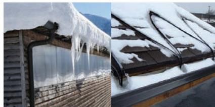
High quality and quick-to-install cable systems for keeping gutters and downspouts free from snow and ice. This heating solution prevents icicle formation and damage to gutters and ensures water can keep flowing freely.
