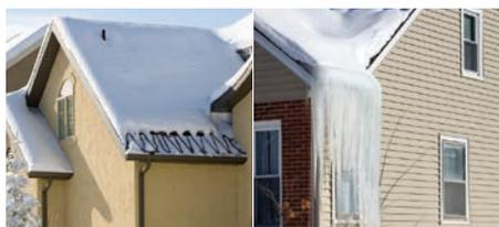
nVent RAYCHEM **roof & gutter de-icing systems** protect roofs and gutters from ice dams, heavy snow build-up and icicles. The heating cable creates a continuous path for melted ice and snow to drain.
