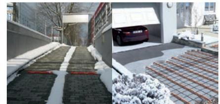
Effective and reliable heating systems for keeping driveways, stairs and footpaths free from snow and ice. This heating solution prevents physical injury and vehicle accidents, and saves time clearing snow.
