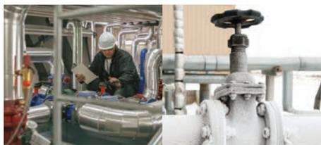
nVent RAYCHEM **pipe freeze protection systems** are flexible and easy to attach to the exterior of the pipe to keep pipes from freezing, bursting, and causing water damage.
