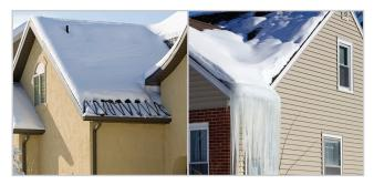
nVent RAYCHEM roof & gutter de-icing systems protect roofs and gutters from ice dams, heavy snow build-up, and icicles. The heating cable creates a continuous path for melted ice and snow to drain.
