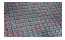
The integrated electric floor heating and uncoupling solution. Membrane can reduce risk of tile cracks due to subfloor movement.
